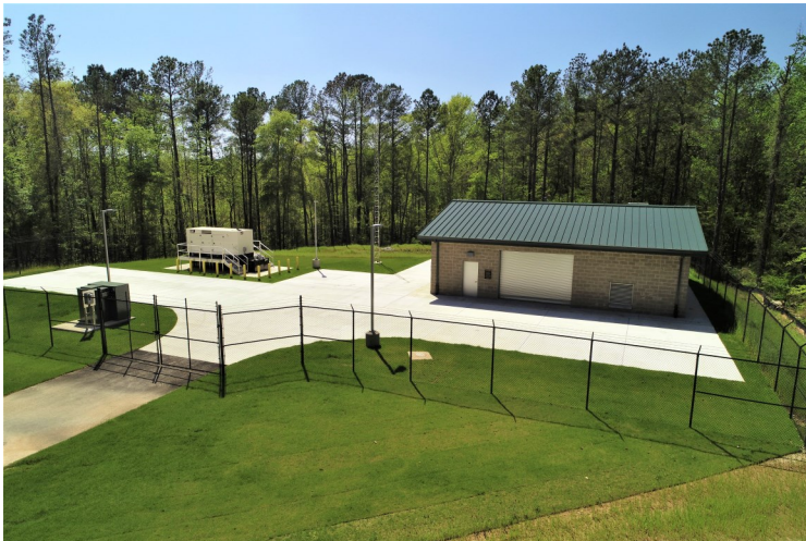
Above: The AWWB's newly constructed Well 4 facility.
